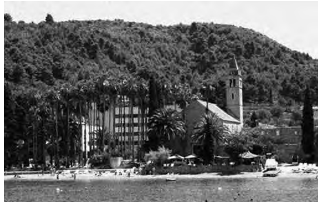
GRAND HOTEL: SHIFTING OF THE REGULATION LINE BEHIND THE EXISTING MONASTERY AND FORMATION OF THE MEDITERRANEAN PARK IN FRONT OF THE BUILDING
