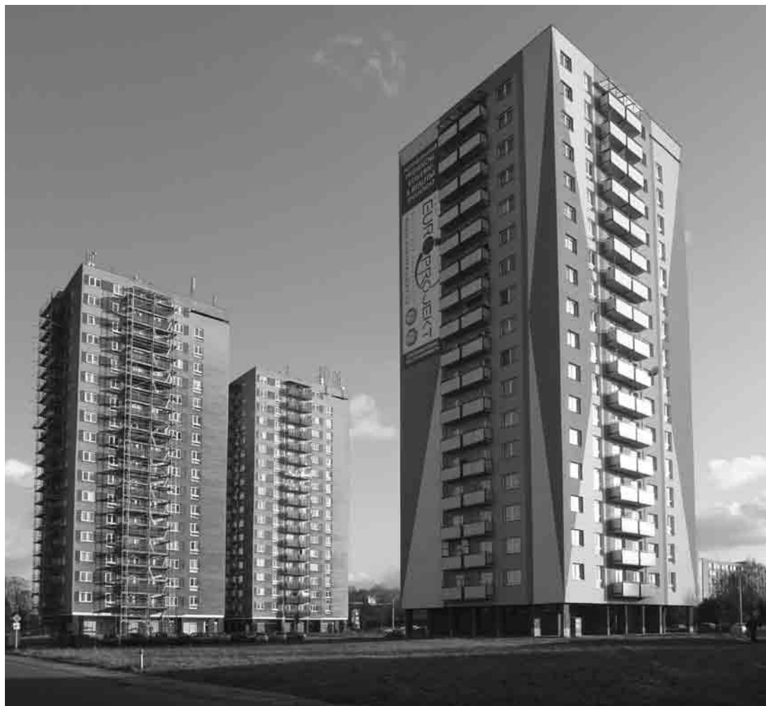
Renovated and unrenovated towers in Ostrava-Zábřeh
