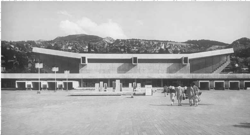
SKENDERIJA, SPORTS CENTRE AND SPORTS HALL BASED ON THE DESIGN OF ŽIVORAD JANKOVIĆ AND HALID MUHASILOVIĆ, 1969
