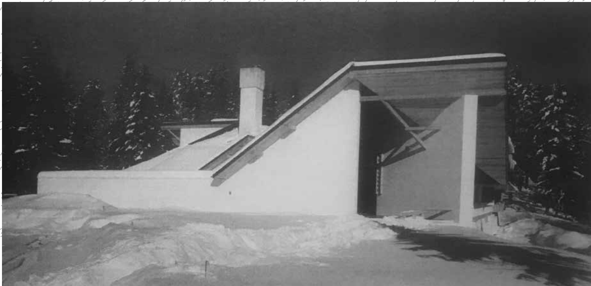
HOTEL VUCKO ON JAHORINA DESIGNED BY ZLATKO UGLJEN, 1984
