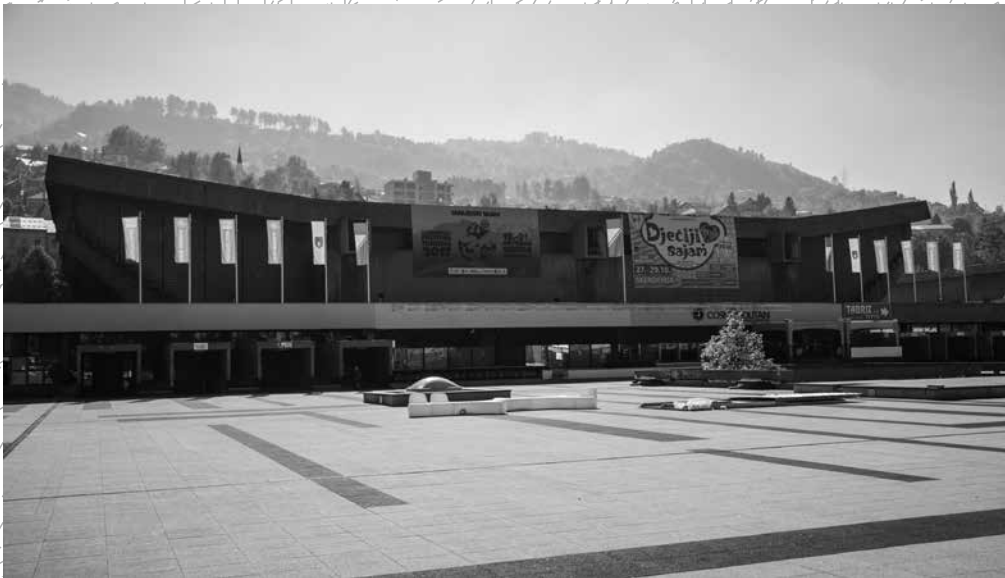
SKENDERIJA, SPORTS CENTRE AND SPORTS HALL BASED ON THE DESIGN OF ŽIVORAD JANKOVIĆ AND HALID MUHASILOVIĆ, 1969
