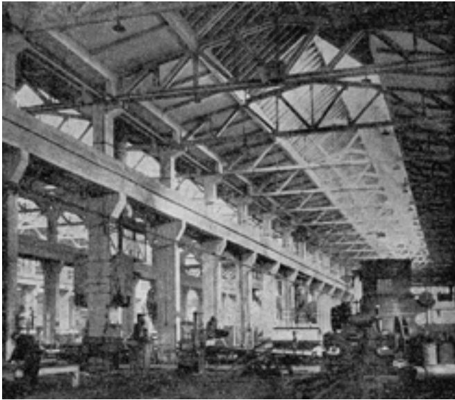
THE "JEDINSTVO" [UNITY] FACTORY IN ZAGREB, INTERIOR OF THE WORKSHOP HALL
