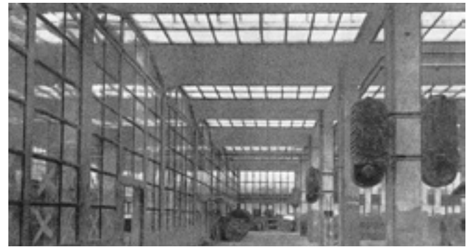
THE JUGOKERAMIKA FACTORY IN POJATNO NEAR ZAGREB, HALL DETAIL
