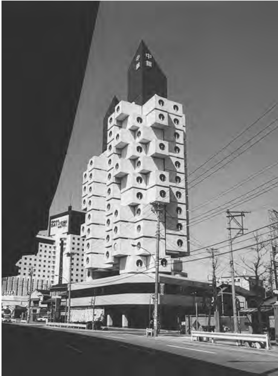
1965, Kurokawa's Nakagin Capsule Tower, composed from two cores with 144 capsules, prefabricated in a factory normally producing shipping containers. With the capsules plugged in and conceived as bolt-holes for homo moven bachelors/commuters, Kurokawa created the dominant icon of Metabolism Source: KUROKAWA, Kisho, 1975. The World of Kisho Kurokawa. Tokyo: Mainichi Newspapers, p. 3.
