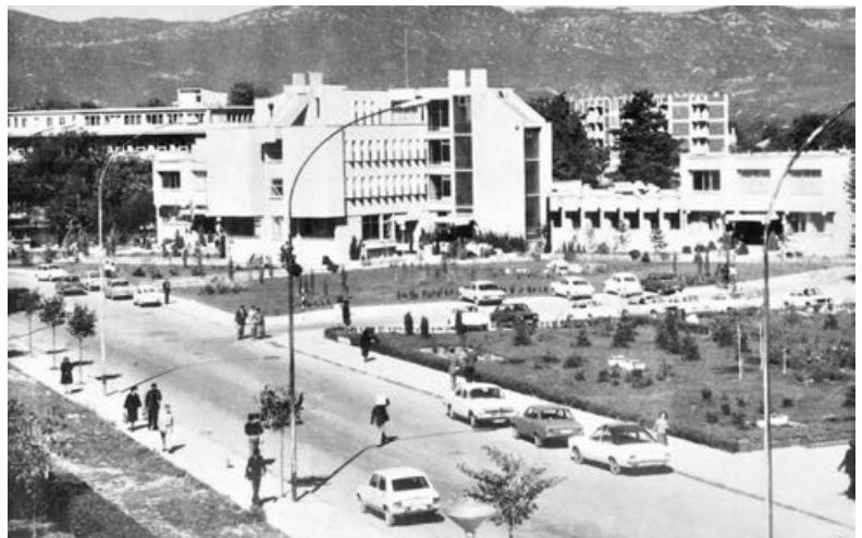
Health Center, architect Dušan Duda Popović, number 9 in the urban ring in the map of locations Source: private archive of Vladimir Bojković
