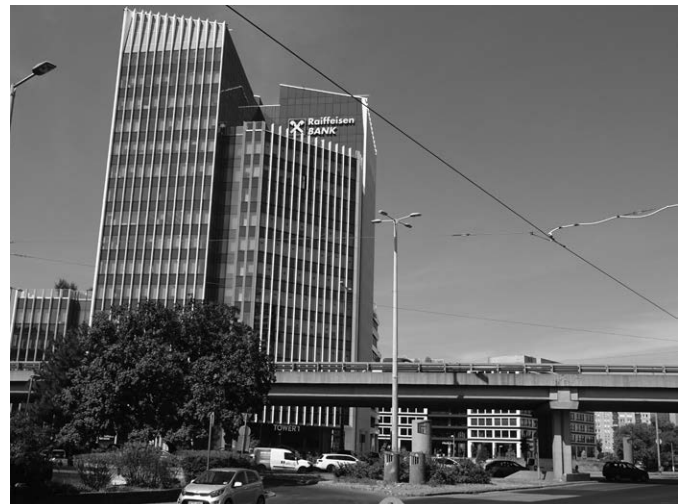
The highest tower of the Agora project with the Váci Street overpass in the foreground in 2024 Photo: Mariann Simon
