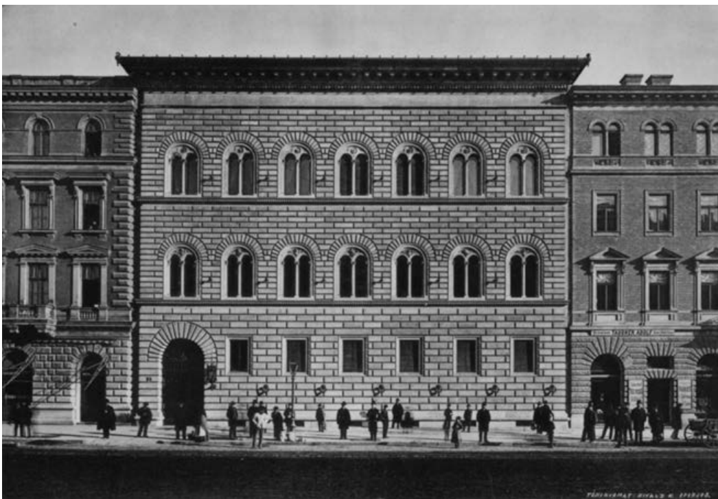
Corner of Ferenc körút and Üllői út; tenement house by József Hubert and Károly Móry, Budapest, photograph, after 1890 Source: Fortepan, photo by György Klösz, inv. no. HU.BFL.XV.19.d.1.07.109, Budapest City Archives
